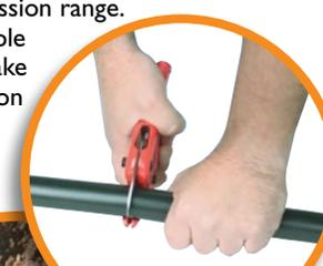
1. Cut the pipe with pipe cutters, knife or saw. Ensure a square cut of pipe ends. Clean burrs from pipe ends. Keep the pipe end clean and as free of scratches and imperfections as possible.
